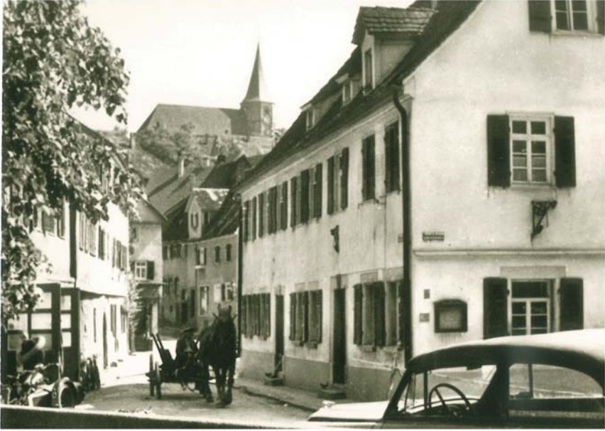
Figure 5: The district prison in which Mrs. Eslinger stayed in 1835/1836 was located on the first floor of the large house in the front. The picture was taken around 1935. It shows the west face of the building and a small part of its south face (compare Figure 2; reprinted with kind permission of the Archiv Stadt Weinsberg ). The five northernmost windows of the first floor belonged to the apartment in which the prison guard and his family lived. The building was demolished in the late 1990s and replaced by a new edifice. The Kernerhaus is located 200m east of the church in the background.
